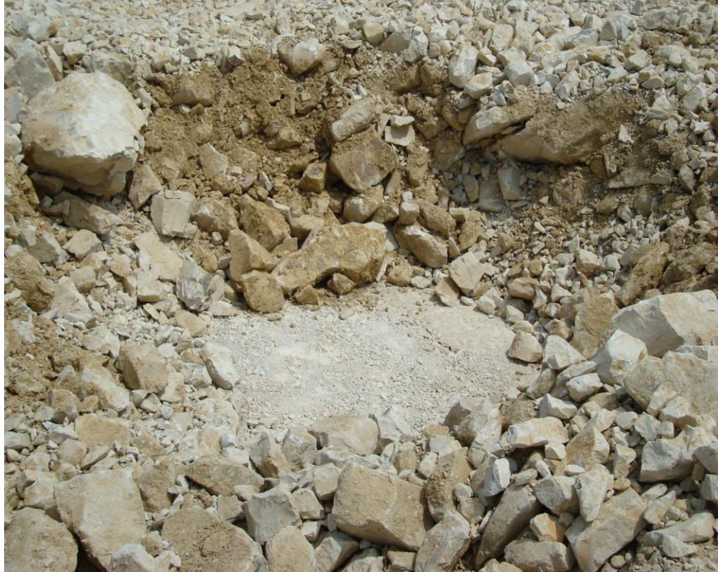
Figure 3.7: The view of Rock Fill after dynamic compaction
