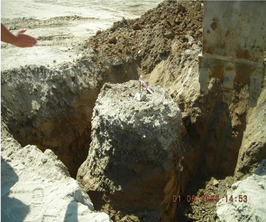
Figure 3.4: Test column with jet-2 method.
