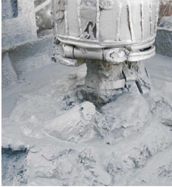
Figure 3.5 Pile drilling Shaft T – coarse silt discharging from the drilling bucket (Martak and Herzfeld, 2005)
