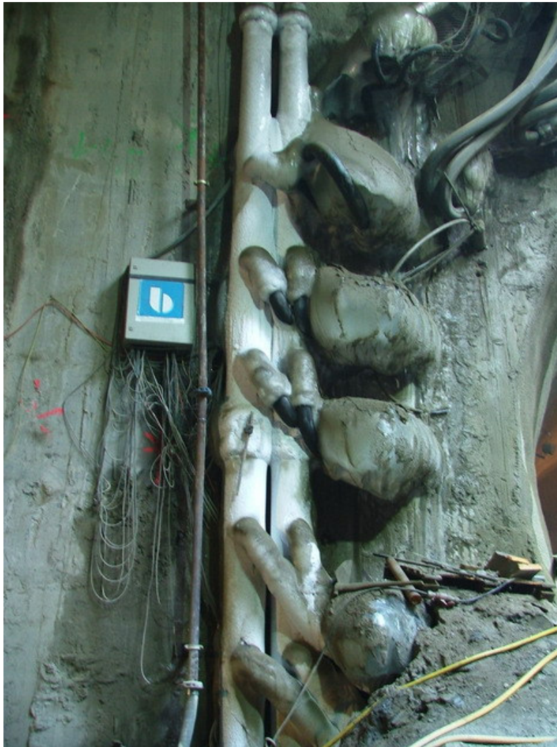
Figure 3.8 Frozen ground after freezing process in U2 Schottenring station
