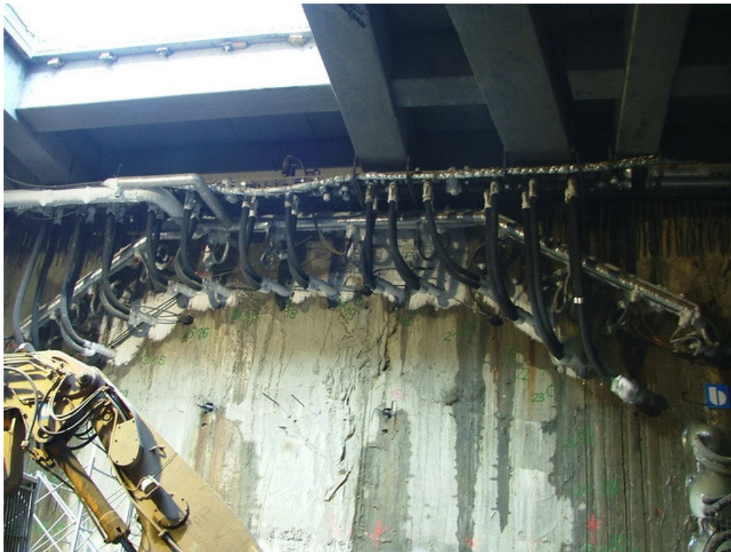
Figure 3.11 Freezing pipes
