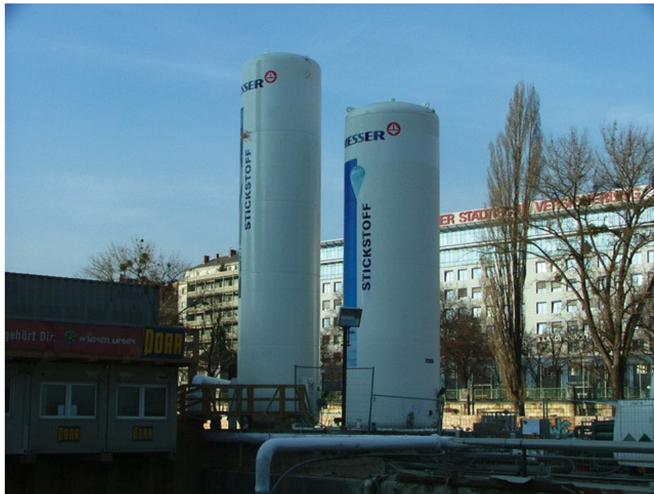
Figure 3.7 Storage tanks of liquid Nitrogen ( \text{LN}_2 )
