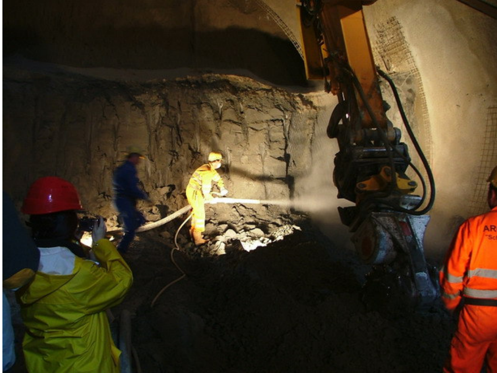
Figure 3.13 Execution of NATM in the construction of U2 Shottenring Station
