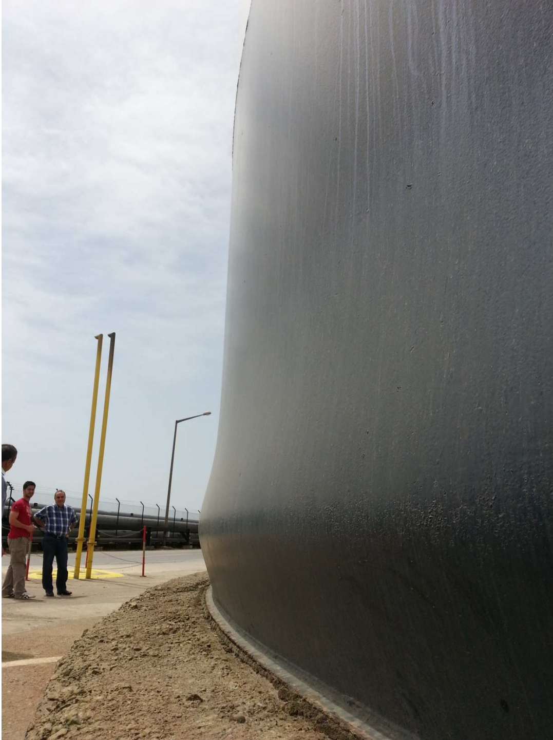
Figure 1.6: Elephant Foot Buckling (TUPRAS, 2013, Personel Picture).
