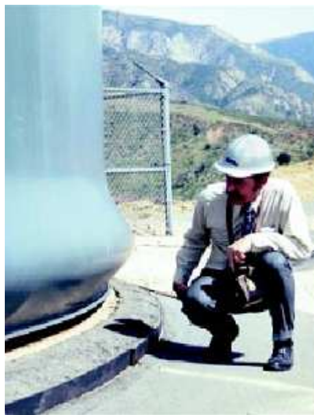
Figure 1.2: Elephant Foot Buckling (Malhotra, 2000).
