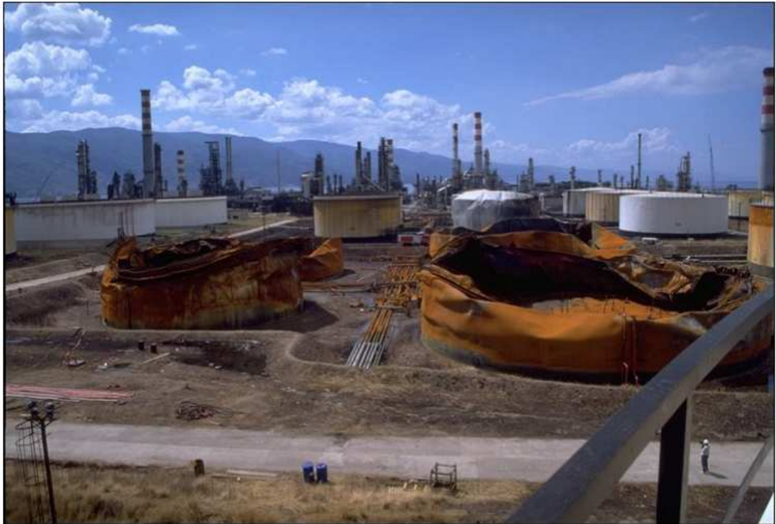
Figure 1.7: Fire Damaged Tanks in Tupras Refinery (Erdik, 2000).
