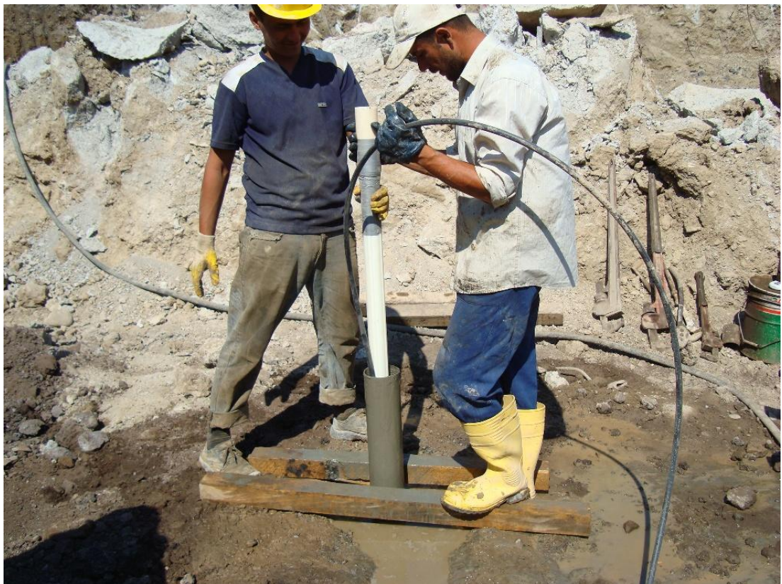
Figure 4.32: Grouting the Well during Installation of the Casings.
