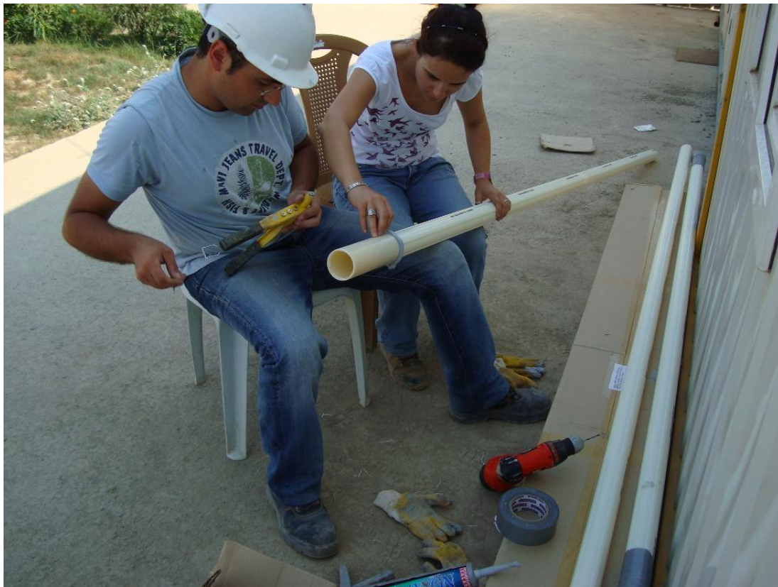
Figure 4.29a: Installation Process Step1.
