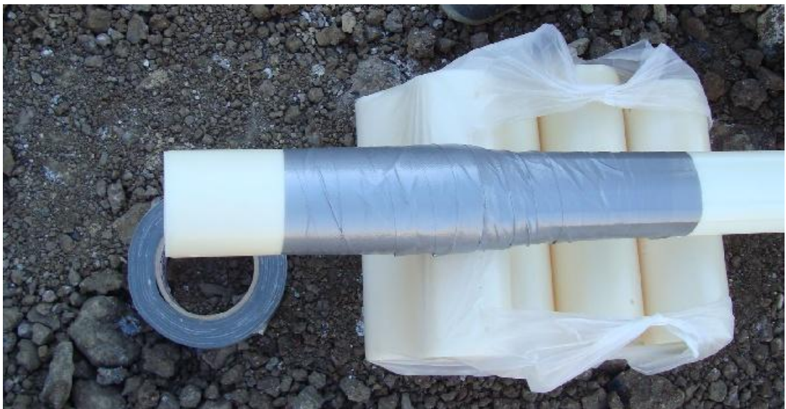
Figure 4.29c: Installation Process Step3.
