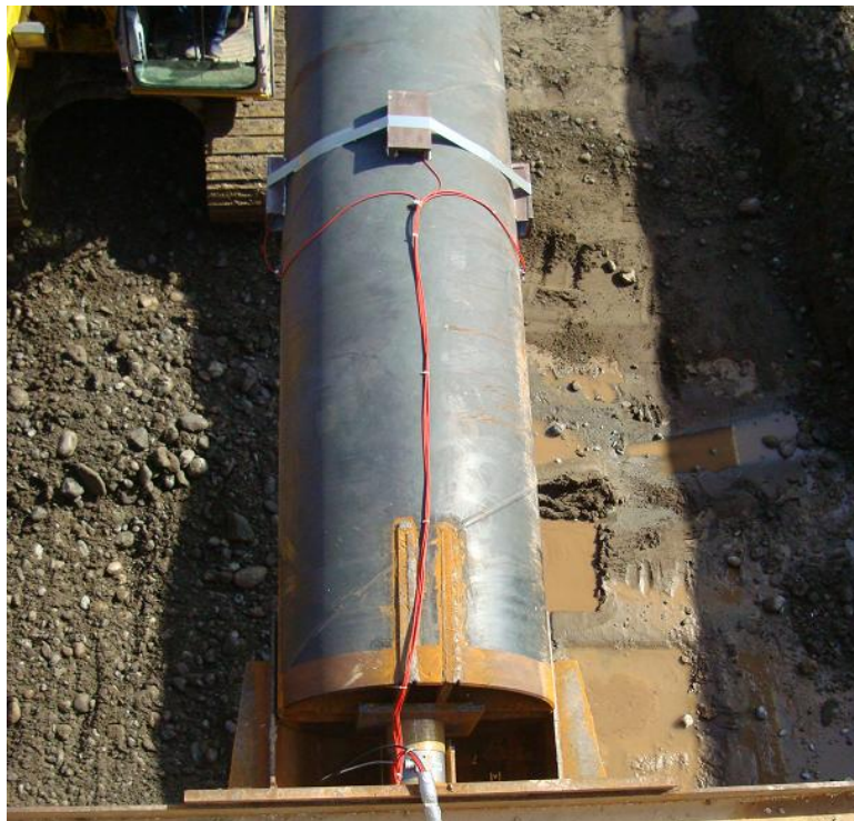
Figure 4.33: Views of Load Cell and Strain Gauges on the Steel Pipe.
