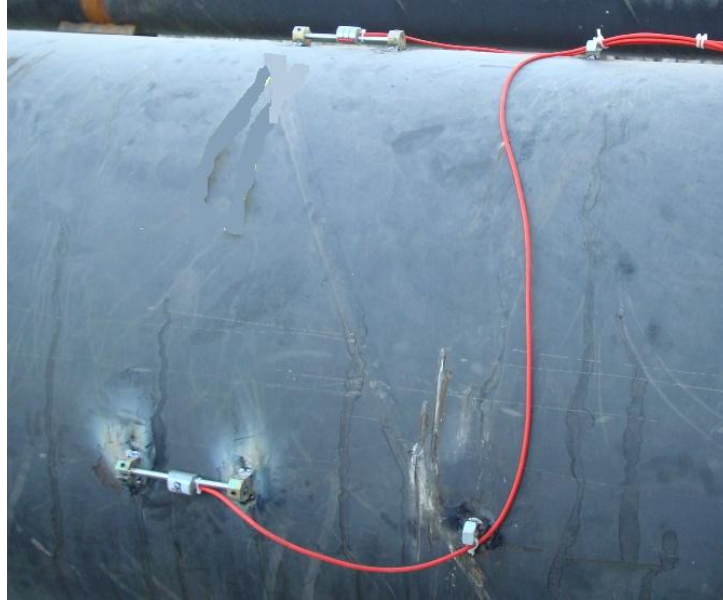
Figure 4.27: Strain Gauges used in the Project.
