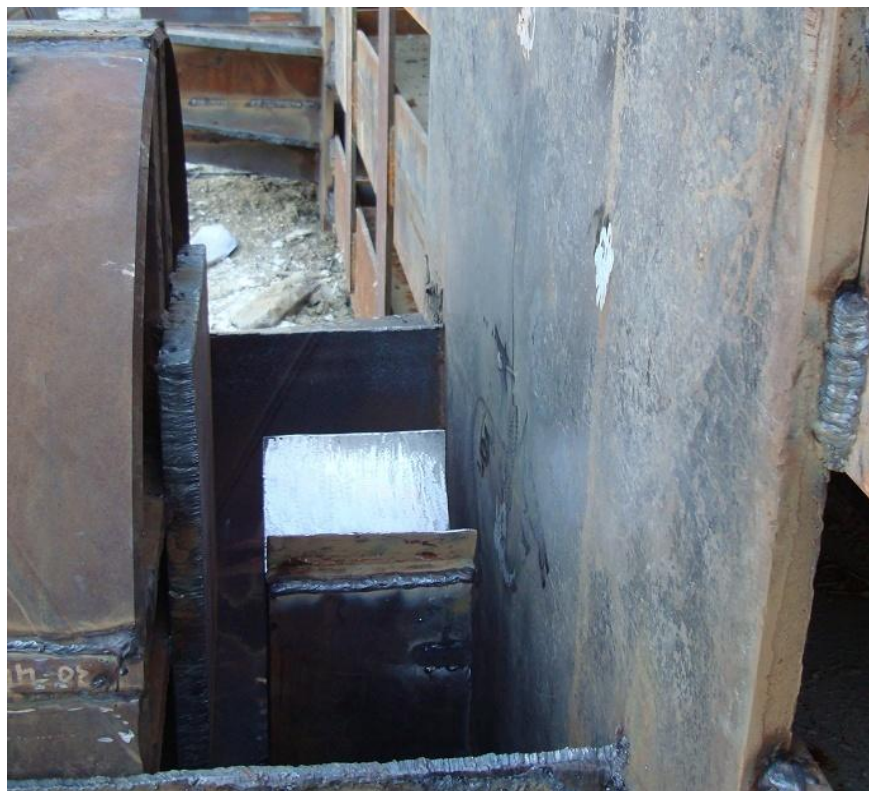
Figure 4.35: Bedding for Load Cell.
