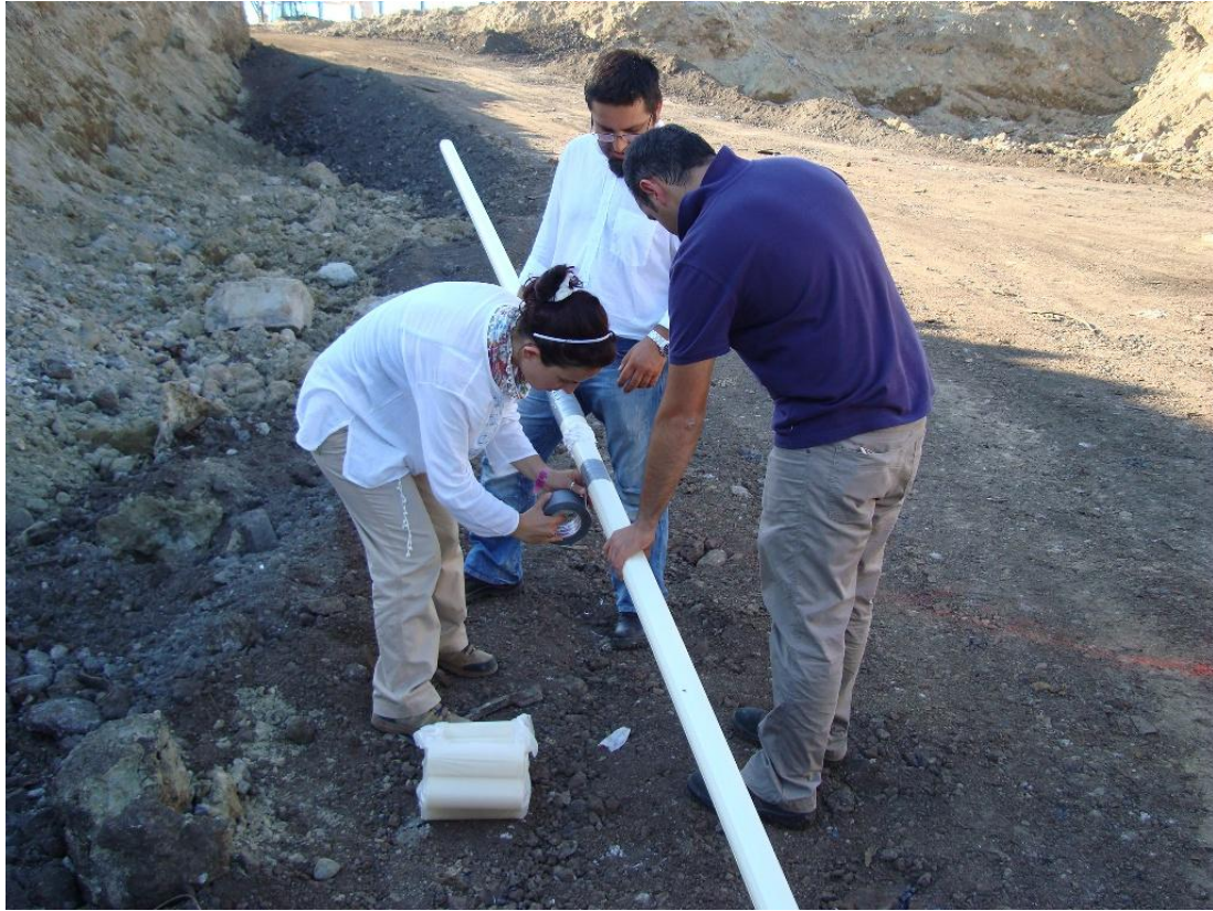
Figure 4.29d: Installation Process Step4.
