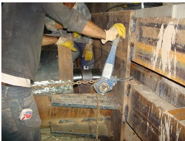
Figure 4.36: Application of the Pre-stress to the Load Cell.
