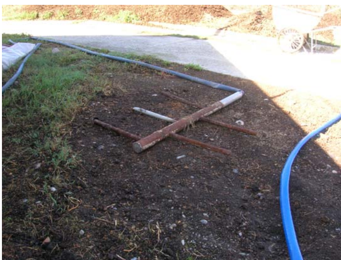
Photograph 3.4. Forced ventilation provided by a perforated pipe
