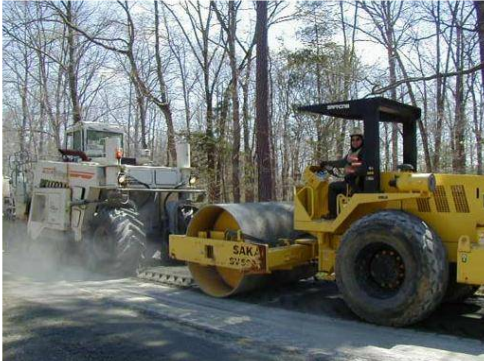
Figure 2.5 : Compaction of the Mixture [2].
