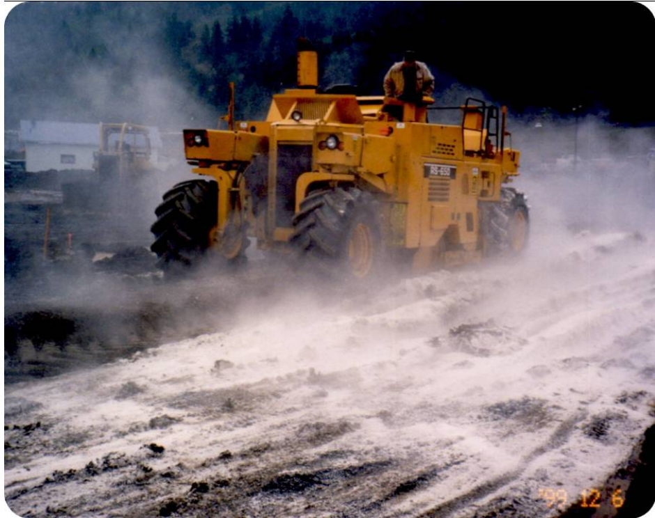
Figure 2.3 : Mixing of the Soil and Additive [2].
