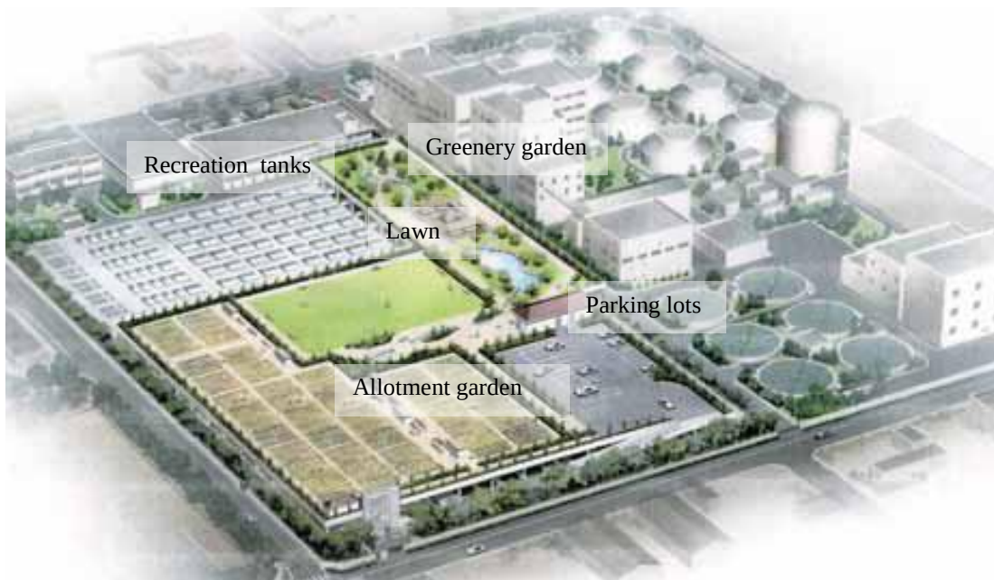
Figure 4.10 : Hanaten Sewage Treatment, full view, after completion (Oono, 2006).
