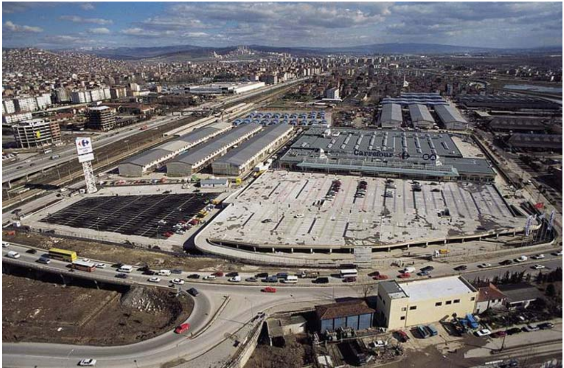
Figure 2.4 : “Shed”: Carrefour, İzmit
