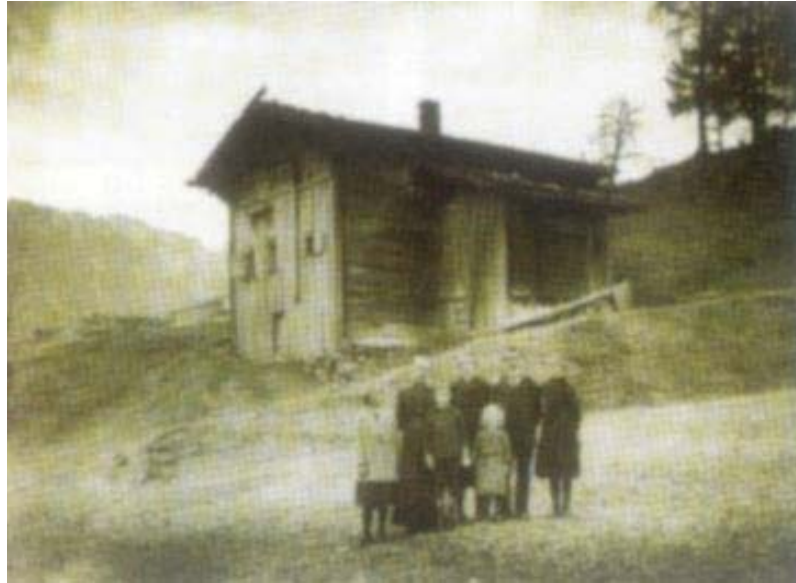
Figure 4.9 : Gugalon House, Graubünden, (Arredamento Mimarlık)
