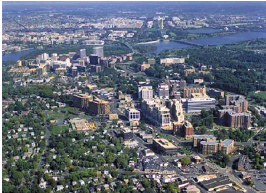
Figure 4.4.1: Aerial view of growth patterns in Arlington County, Virginia (Internet)
