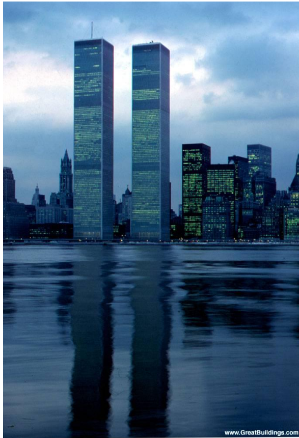
Figure 3.2.6: The World Trade Center (Twin Towers) in New York (Internet)
