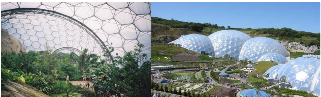
Şekil 2.13: Eden Project, 2003, Grimshaw Architects (Pawlyn, 2011).
