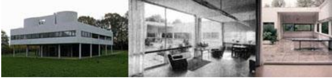
Resim 3.7. Villa Savoye, Poissy-Fransa, Le Corbusier, 1930. ( kaynak: http://www.greatbuildings.com/buildings/Villa_Savoye.html (sol), http://www.arkitera.com/diyalog/ihsanbilgin/lecorbusier.htm (orta), Tzonis, A., 2001. Le Corbusier The Poetics of Machine and Metaphor , Thames and Hudson, London, s. 66. (sağ))
