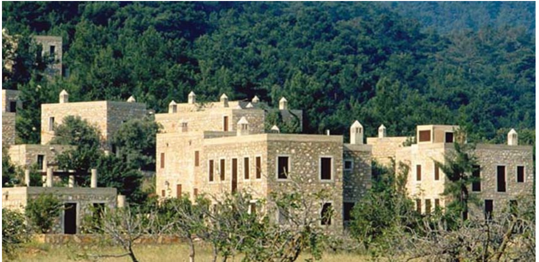
Şekil 4.15: Demir Evleri, genel görünüş (Aga Khan Award for Architecture, http://archnet.org/library/images/one-image.tcl?location_id=2409&image_id=74548 )
