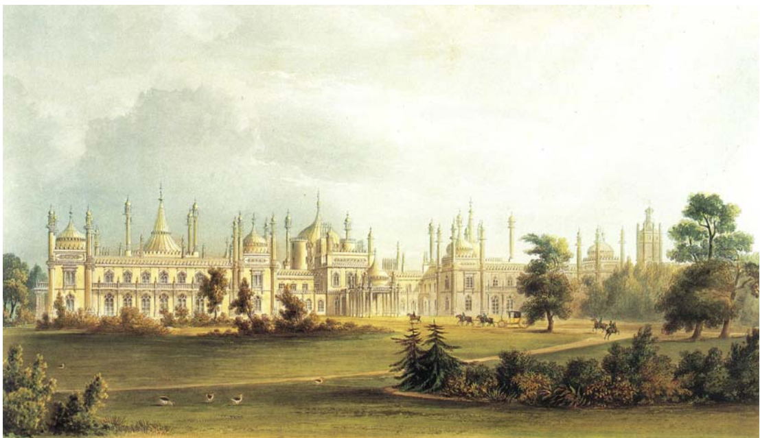
Figure 5.2.3- 16 John Nash: The west façade of the Royal Pavilion, 1823 [38, p. 41].
