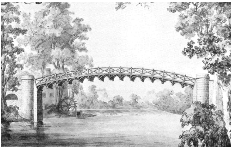
Figure 5.2.3- 2 John Nash: The iron bridge at Stanford-on-Teme, Worcestershire, 1795 [48, PLATE 4B].
