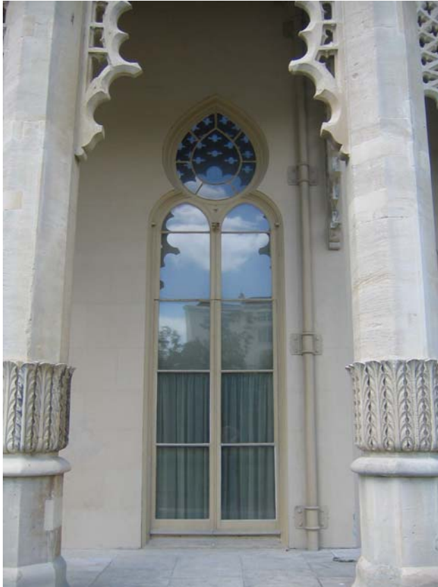
Figure 6.3.1- 7 East façade: Detail from the French windows [Original].
