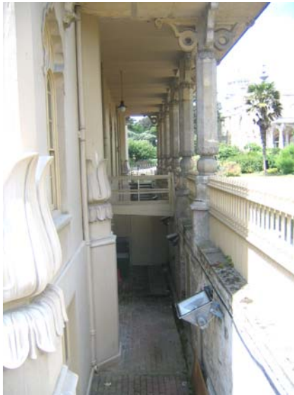
Figure 6.3.2- 4 North façade: Lateral view [Original].
