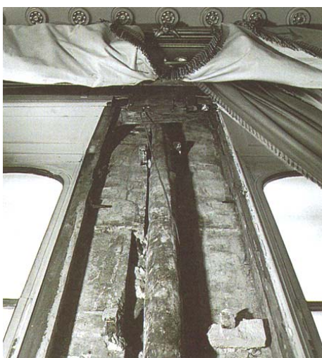
Figure 6.2- 5 Detail from an internal rainwater drainpipe [56, p. 40].
