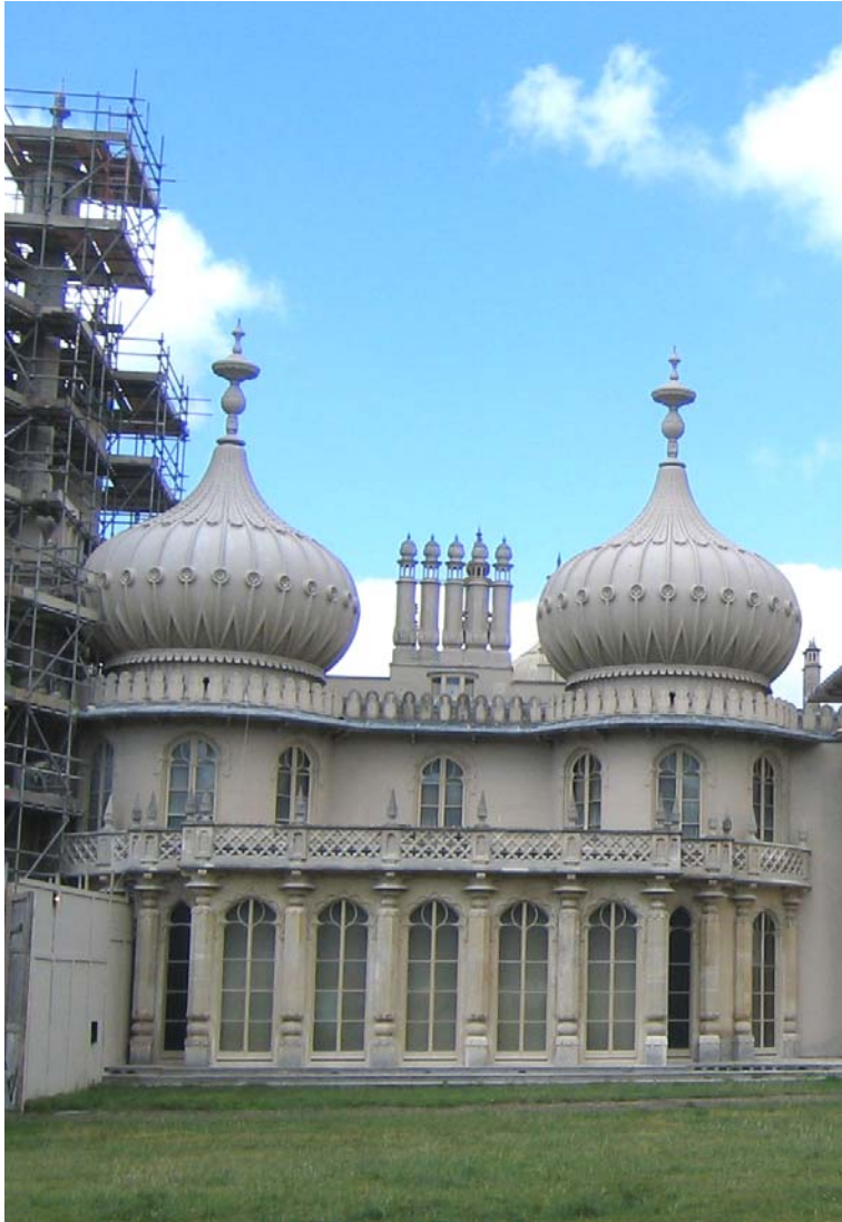
Figure 6.3.1- 3 East façade: One of the horizontal wings on both sides of the rotunda [Original].
