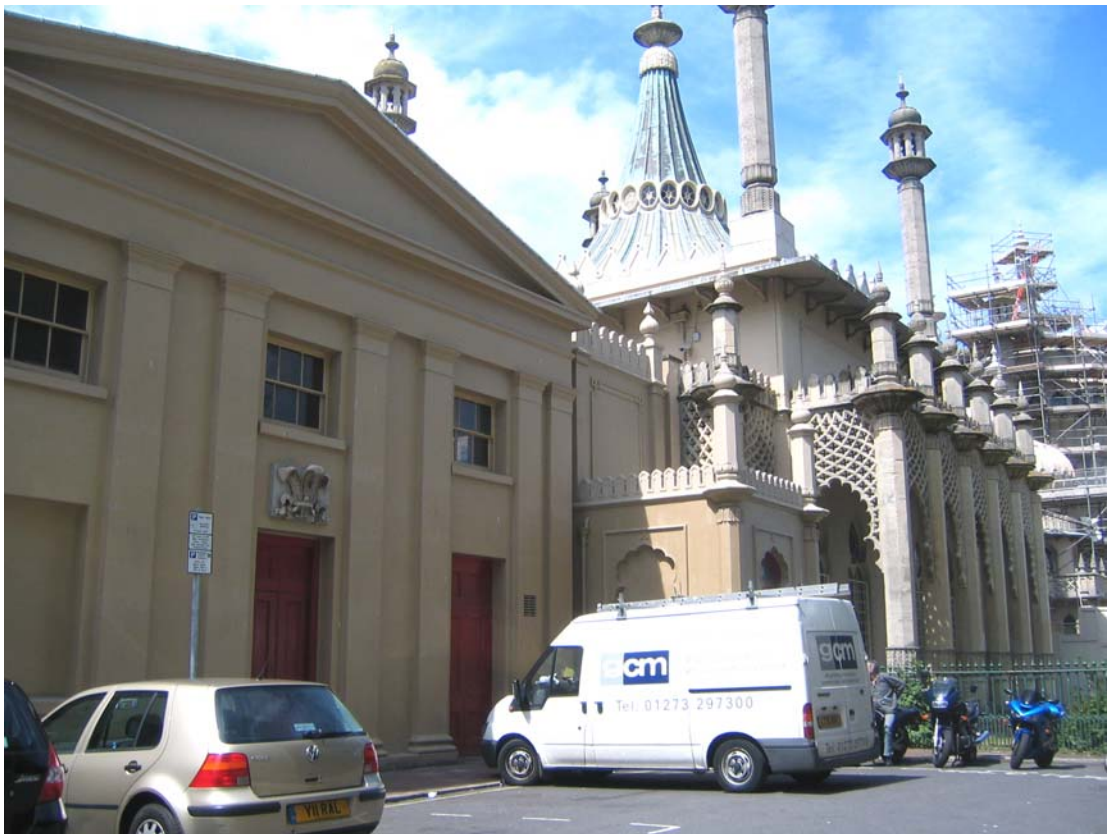
Figure 6.3.1- 12 East façade: The kitchen block at the south end [Original].
