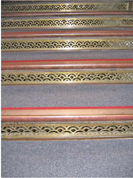
Figure 6.4.1.3- 9 The Long Gallery: Detail of the cast-iron staircases [Original].
