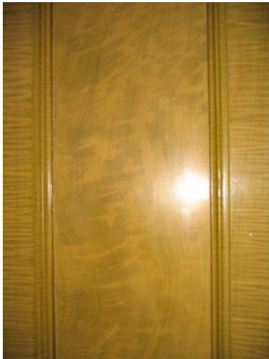
Figure 6.4.1.10- 5 The King's Library: Detail of the graining of the doors [Original].
