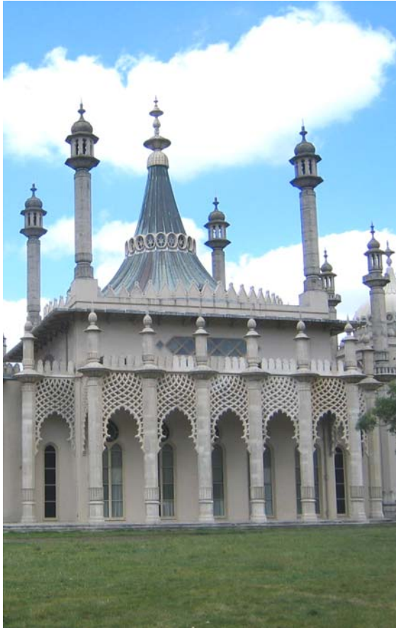
Figure 6.3.1- 5 East façade: One of the main State Rooms on each end [Original].
