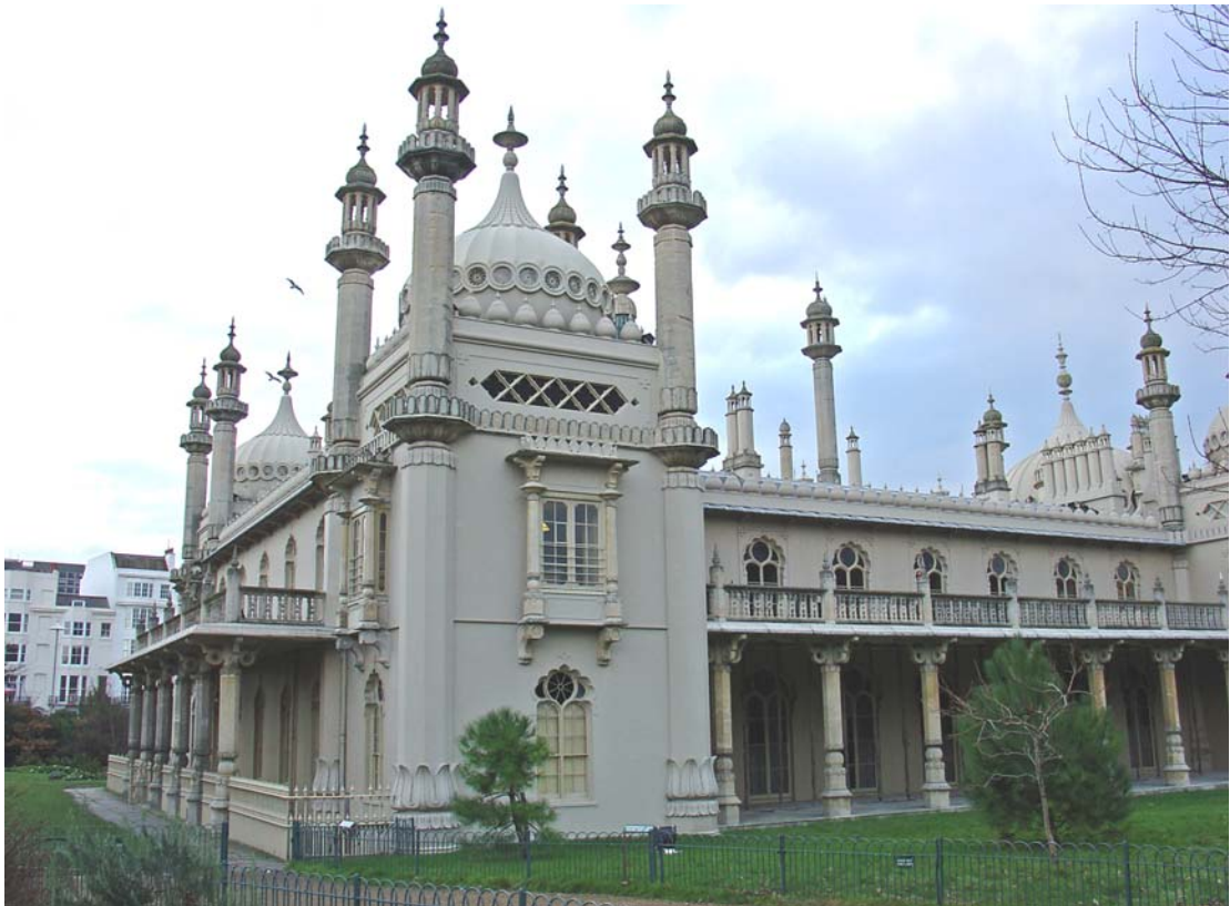
Figure 6.3.3- 1 Perspective view of the north-west façades of the Royal Pavilion [Original].
