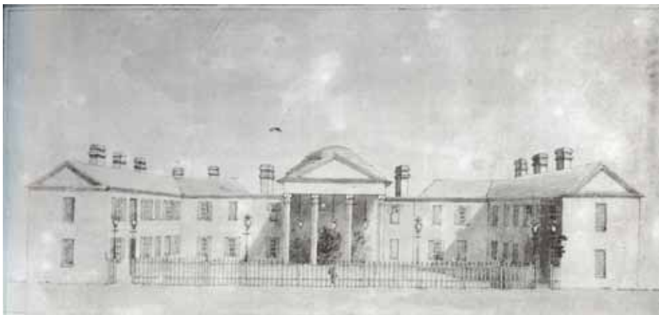
Figure 5.2.1- 6 Henry Holland: West façade of the Marine Pavilion, 1788 [41, p. 31].
