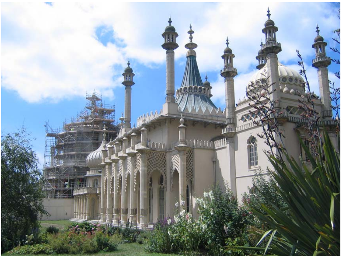
Figure 6.3.1- 8 East façade: Perspective view of the tower block at the north end [Original].
