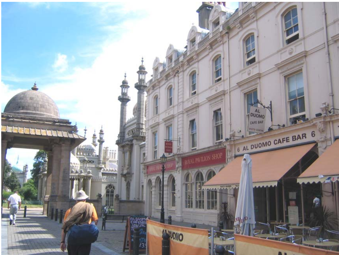
Figure 6.3.3- 4 West façade: View of the blocks attached to the Royal Pavilion from the south end [Original].
