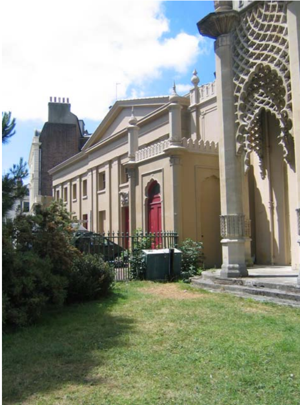
Figure 6.3.1- 11 East façade: The kitchen block at the south end [Original].
