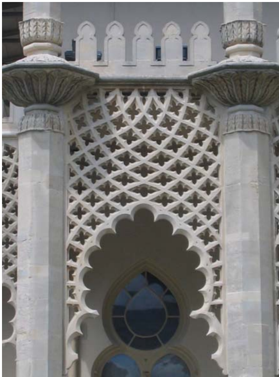
Figure 6.3.1- 6 East façade: Detail from the perforated stone screens [Original].
