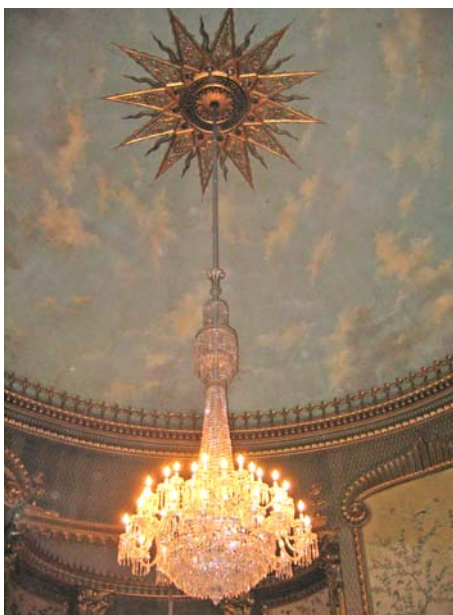
Figure 6.4.1.8- 5 The Saloon: Detail of the ceiling [Original].
