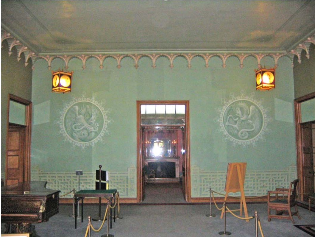
Figure 6.4.1.2- 5 The east wall of the Entrance Hall [Original].
