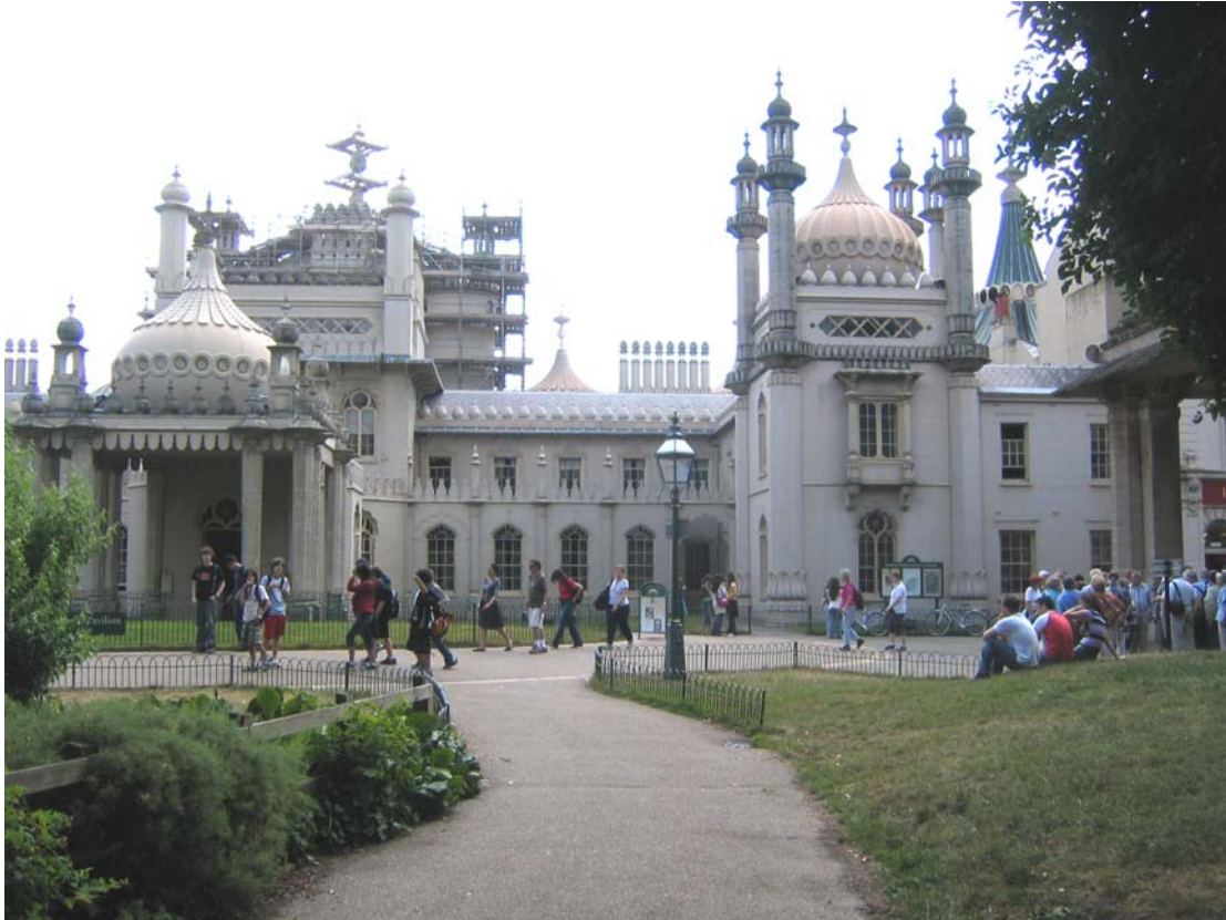
Figure 6.3.3- 3 West façade: Detail view from the south end [Original].
