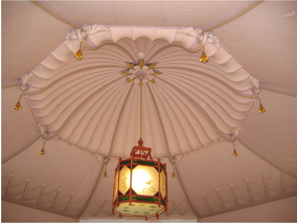
Figure 6.4.1.1- 3 The Octagon Hall: Ceiling detail [Original].
