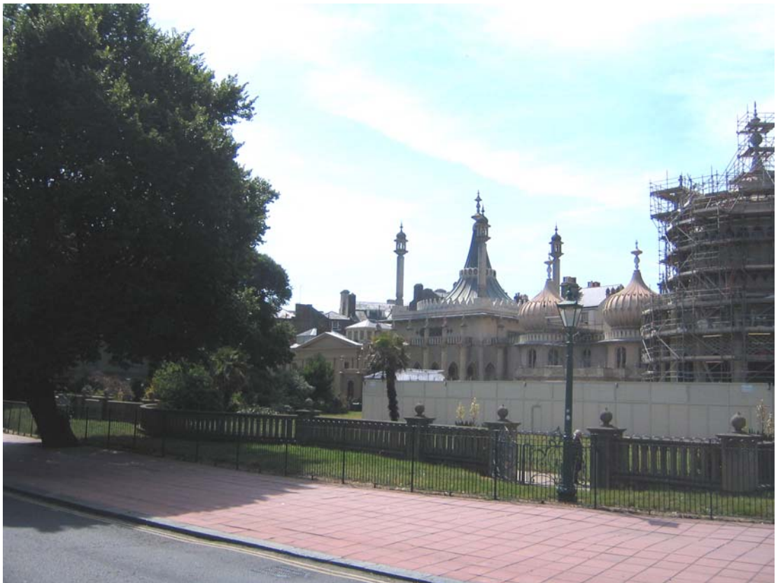
Figure 6.3.1- 10 East façade: View from the Steine, depicting the kitchen block at the south end [Original].
