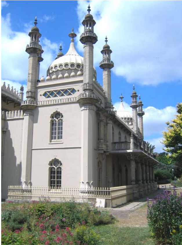
Figure 6.3.1- 9 East façade: The tower block at the north end [Original].
