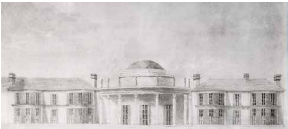
Figure 5.2.1- 5 Henry Holland: East façade of the Marine Pavilion, 1788 [41, p. 30].
