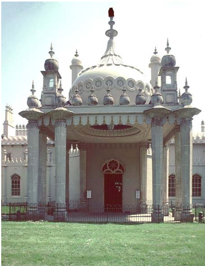
Figure 6.3.3- 6 West façade: View from the main entrance [86].
