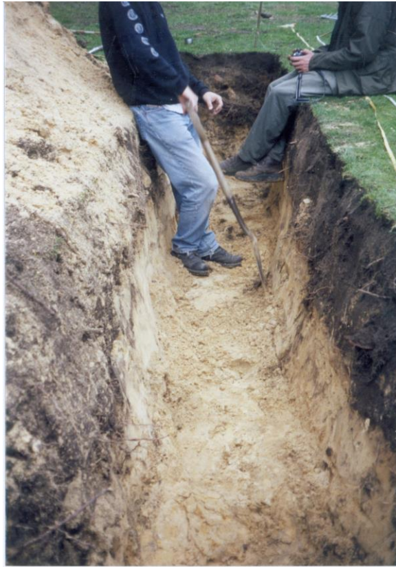
Figure 3.4. Excavated area in the test field.
