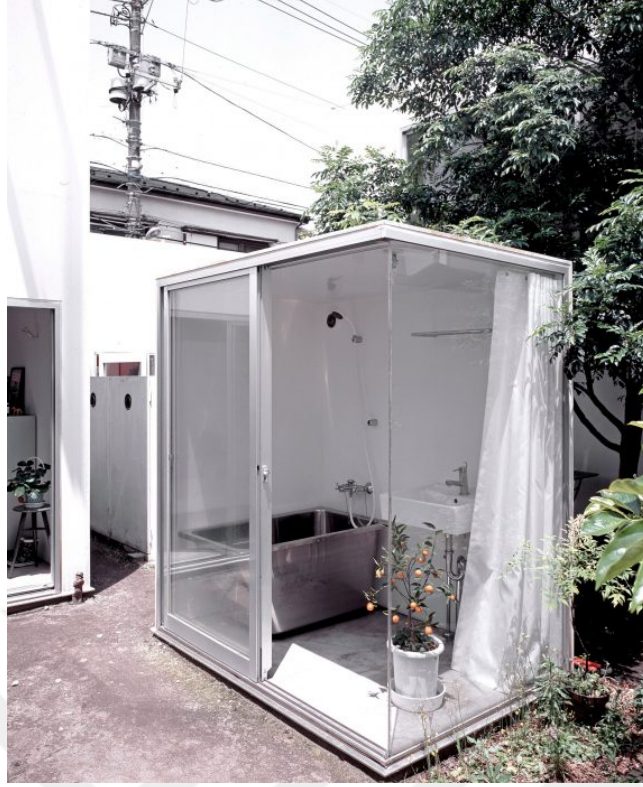
Şekil 2.1.8: SANAA / Kazuyo Sejima + Ryue Nishizawa, Moriyama House, 2011.
