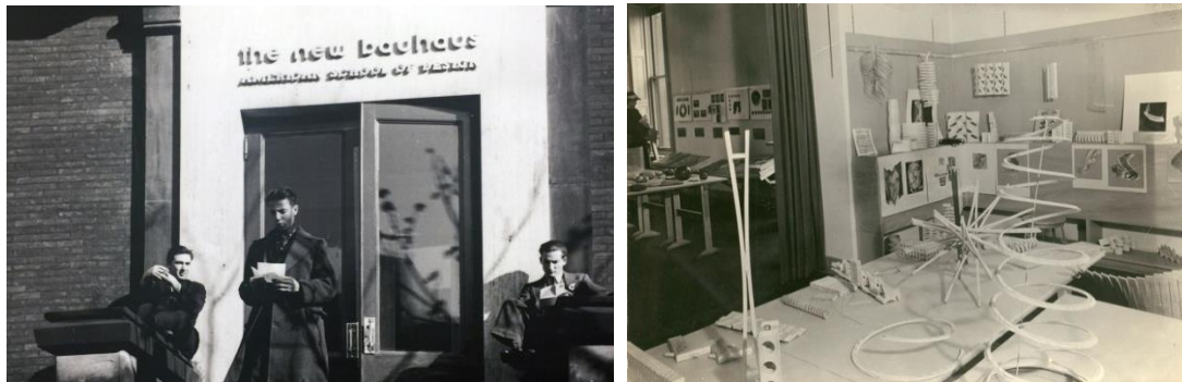
Figures 3.5 and 3.6 : Exterior view of the “New Bauhaus” and the exhibition of student work from the preliminary course (Marshall Field mansion, 1927-1938)
