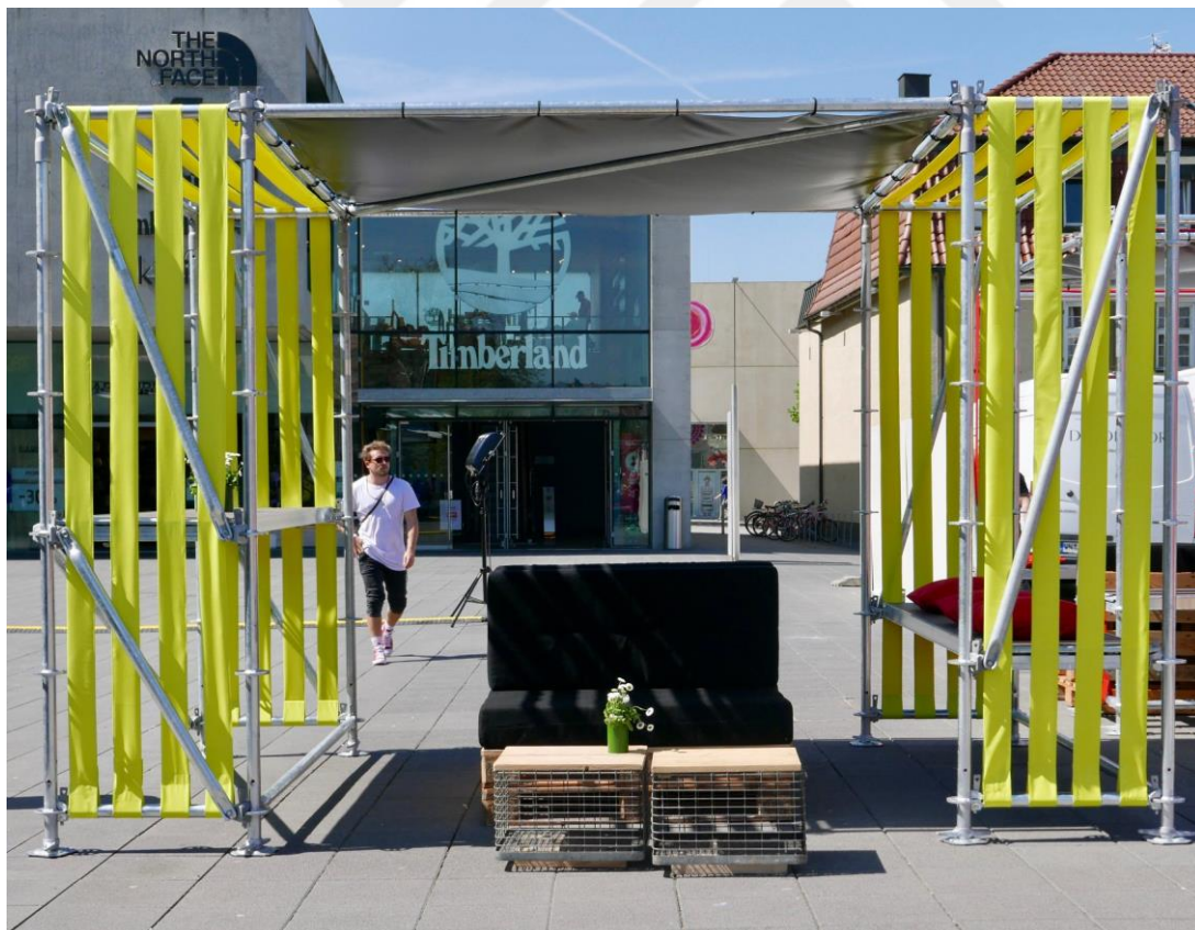
Figure 4.11 : D+M's scaffold structure module with yellow textile (URL-9).
