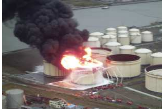
Figure 1.15 : Fire in oil tanks after the 2003 Tokachi-oki earthquake (Url-17).
