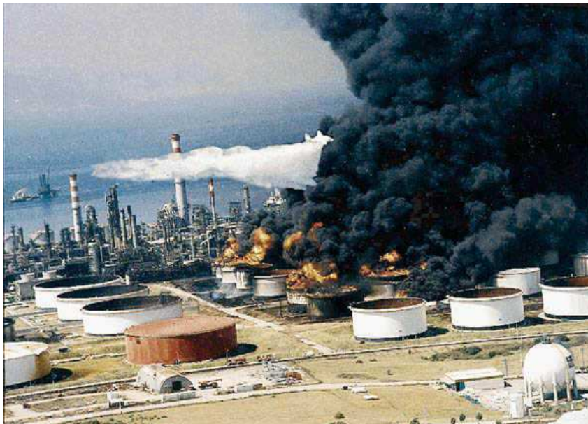
Figure 1.14 : Fire in tanks following the 1999 Marmara earthquake (Url-16).
