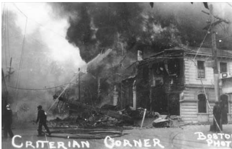
Figure 1.5 : A view of Criterion Corner in the 1931 Napier earthquake (Url-6).
