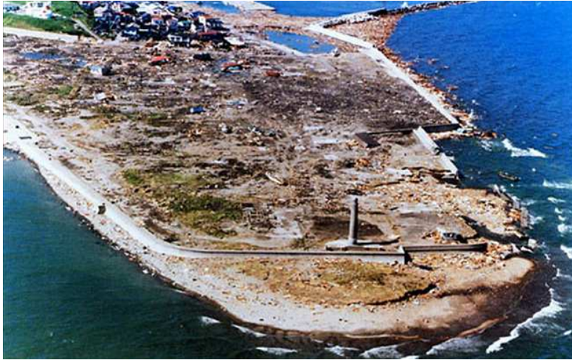
Figure 1.10 : Aonae area of the island Okushiri after the 1993 Hokkaido Nansei-oki earthquake (Url-12).
