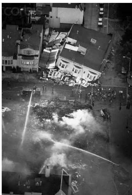
Figure 1.8 : Marina District Fire in the 1989 Loma Prieta earthquake (Url-9).
