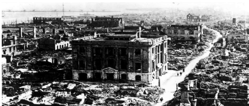
Figure 1.3 : Destruction of Tokyo due to the quickly spreading fires following the 1923 Great Kanto earthquake (Url-4).
