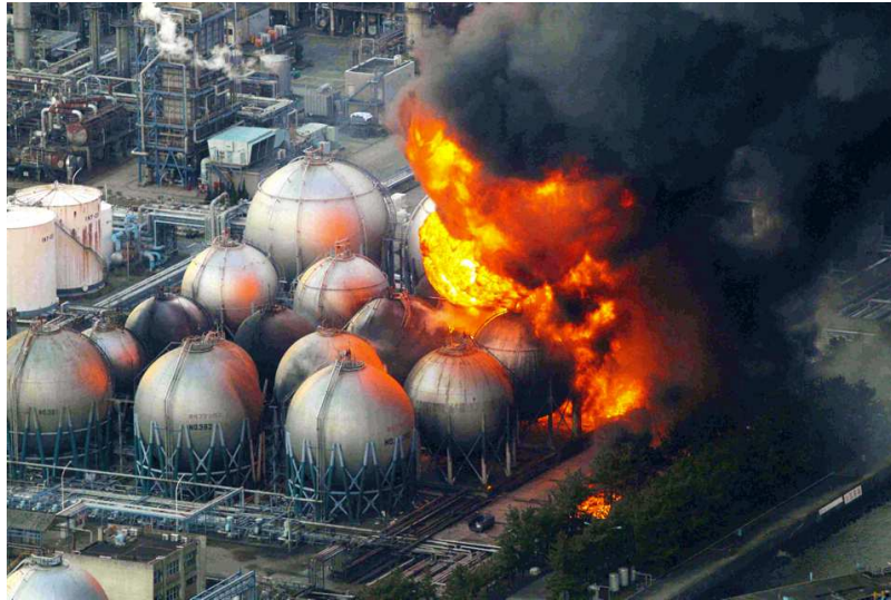
Figure 1.17 : An oil refinery is on fire following the Tohoku earthquake in Chiba city, Chiba prefecture (Url-19).
