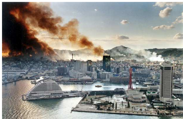
Figure 1.13 : Aerial photograph of Kobe City in the 1995 Hyogo-ken Nambu earthquake (Url-15).
