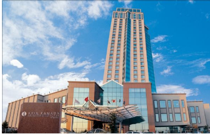
Şekil 4.8 : Kaya Ramada Otel, İstanbul ( http://wyndhamworldwide.com , 2009).
