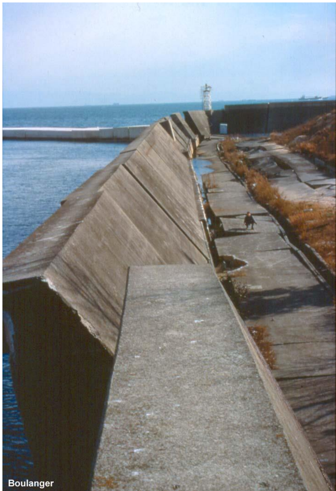
Figure A.5: Quay wall along channel.
