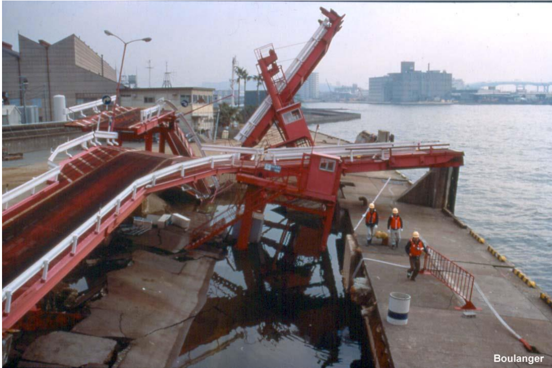
Figure A.3: Ferry ramp collapse.
