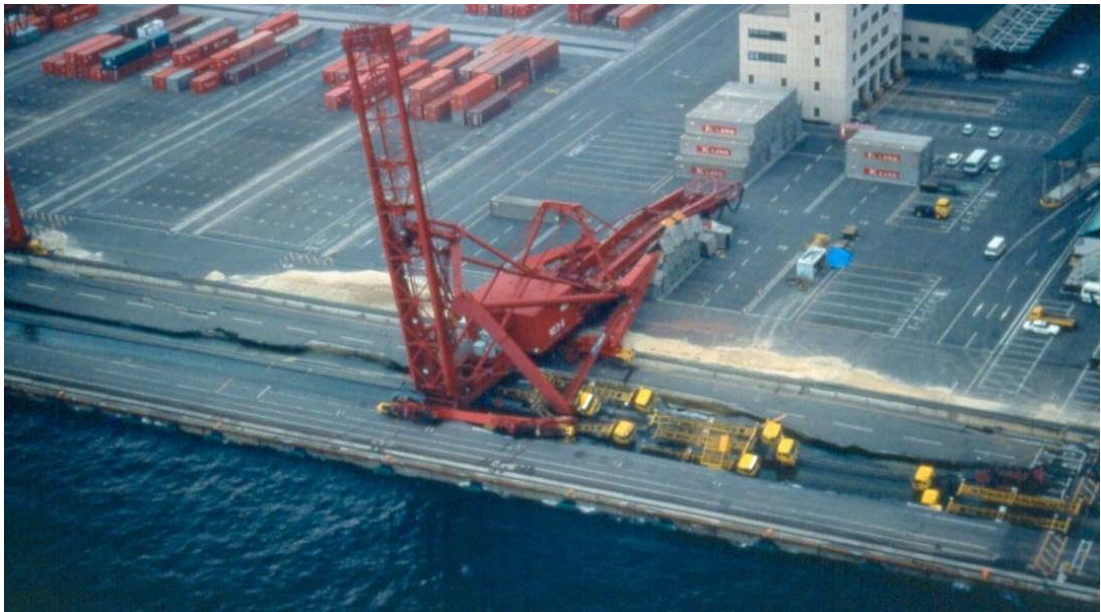
Figure A.1: Aerial photograph of collapsed crane.
