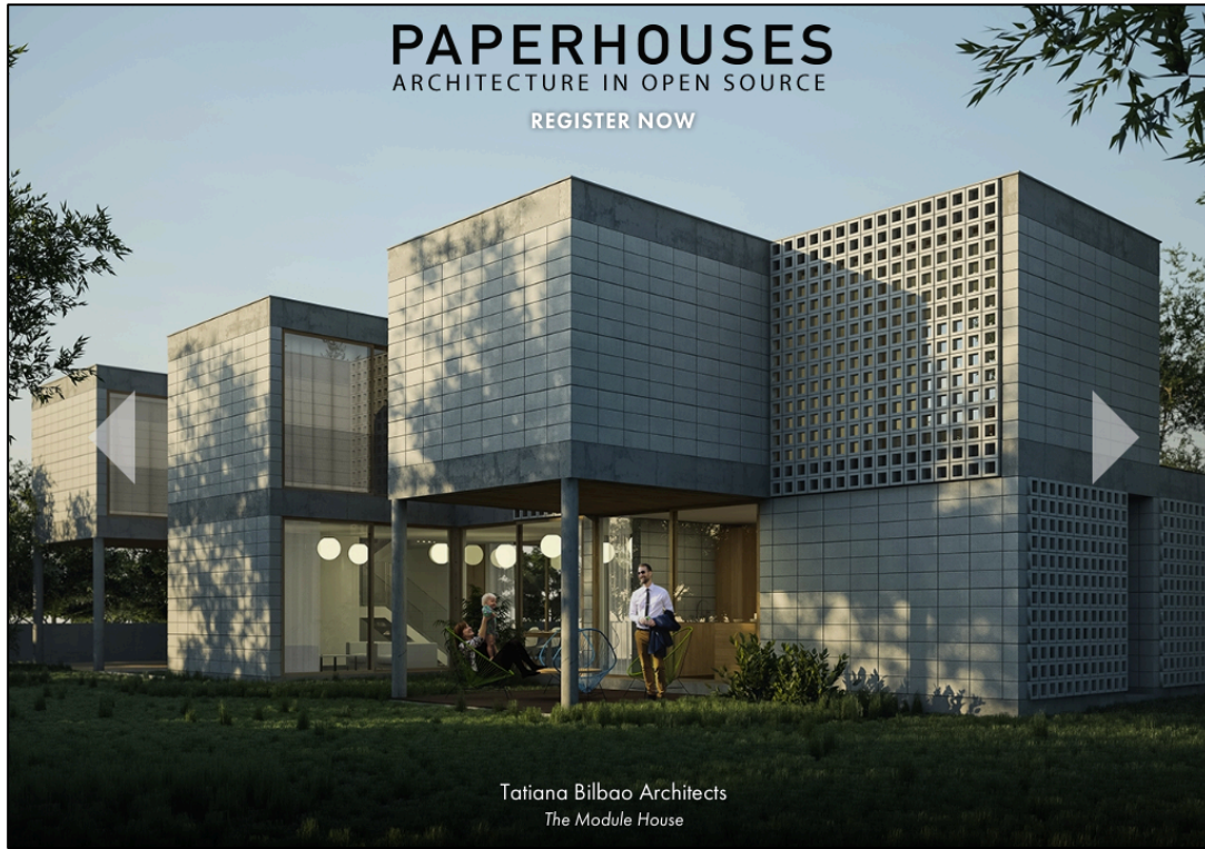
Şekil 3.16: The Module House (Paperhouses, 2014).
