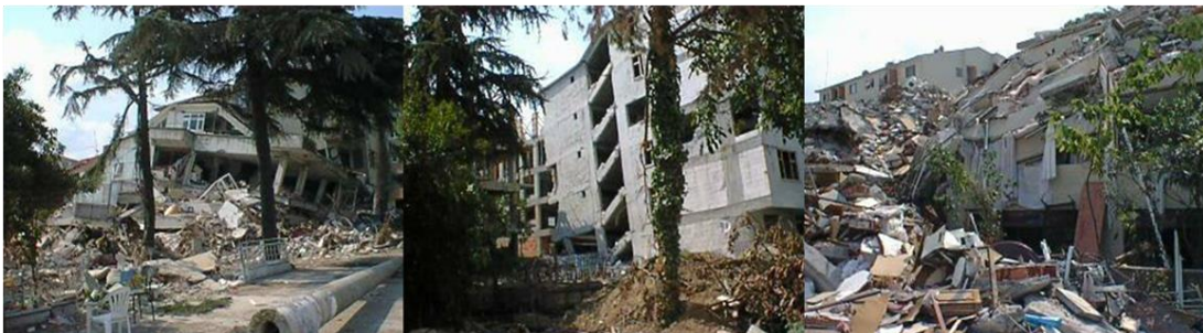
Figure 2.4 : Collapsed buildings photo from Gölcük.
