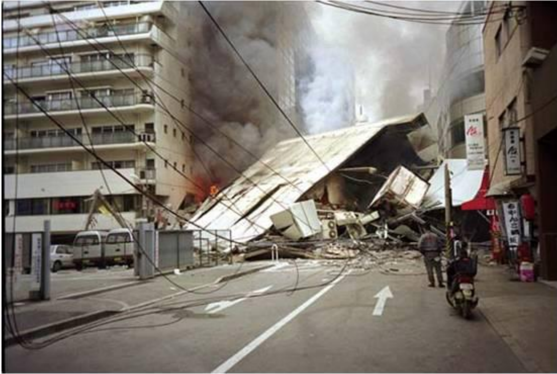
Figure 2.3 : Road blockage due to the building collapse from 1995 Kobe Earthquake, (2015).
