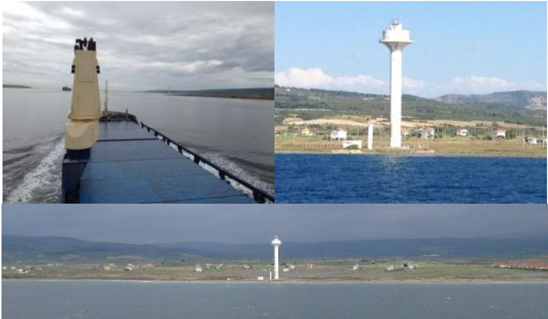
Figure 2.50 : Gocuk Burnu Light and VTS radar tower.
