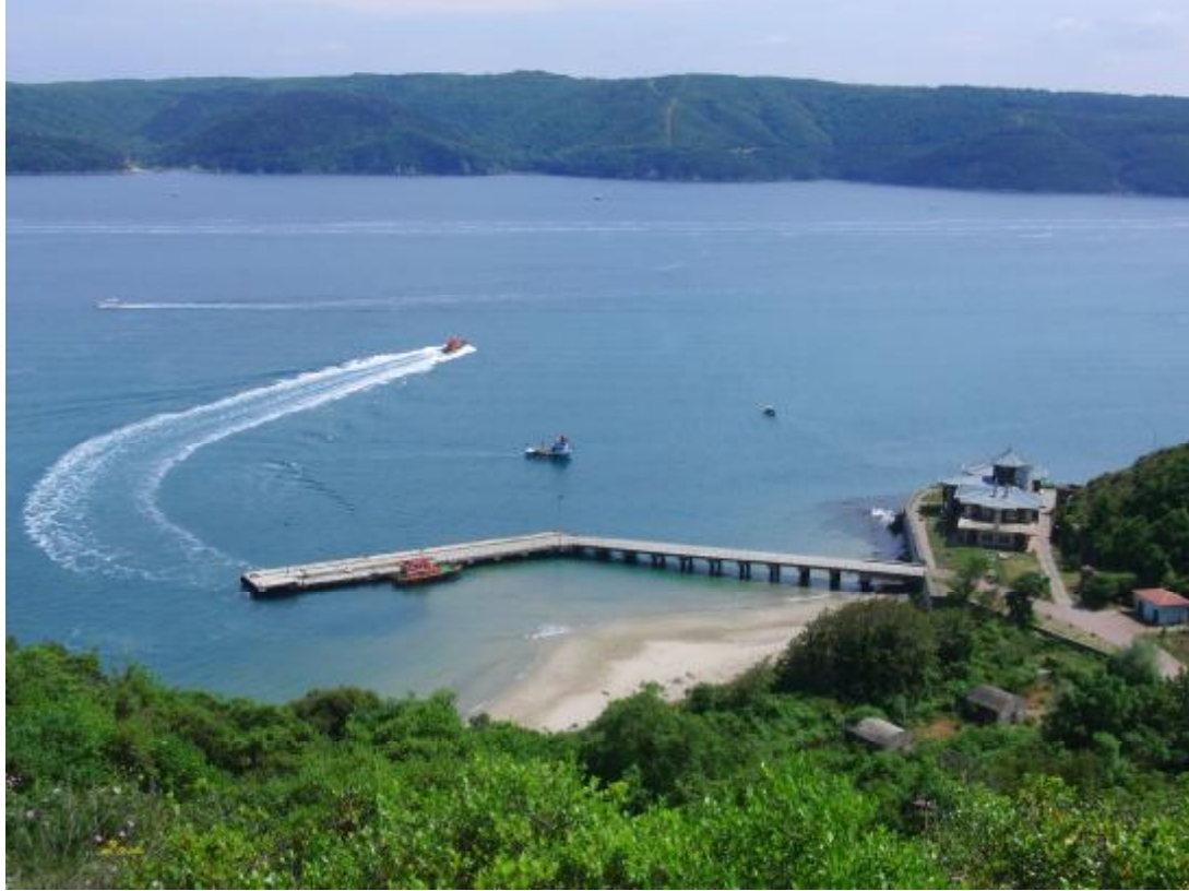
Figure 2.4 : Kaptan Lütfü Berk Pilot Station.
