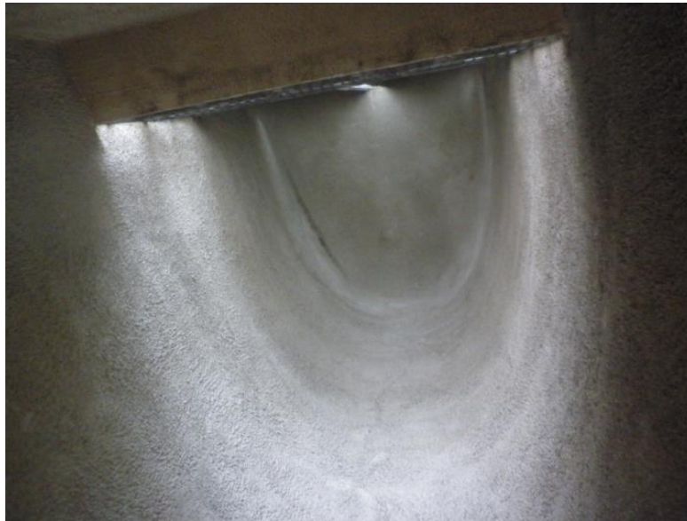
Figure 5. 65 : Interior view of west facing light scoop ( Gültekin, 2014).
