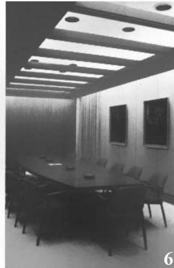
6. Lighting of cove above, Lighting of walls flat shadow free
