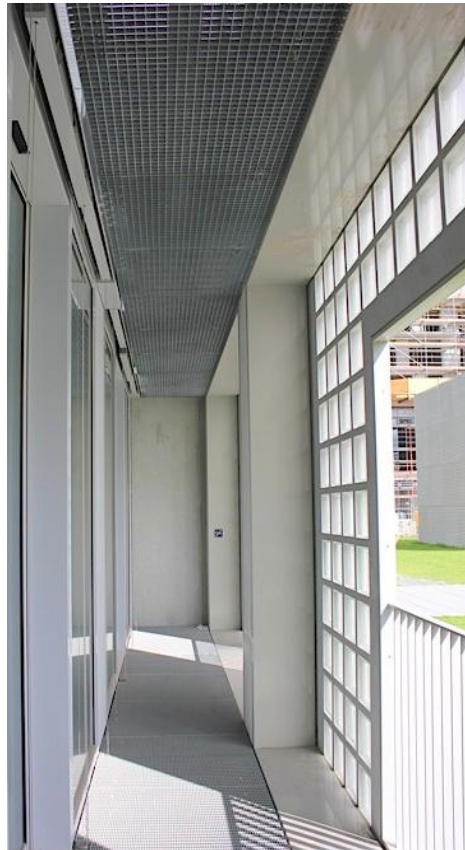
Figure 5.16 : The corridor formed in between two facades (Gültekin, 2014).
