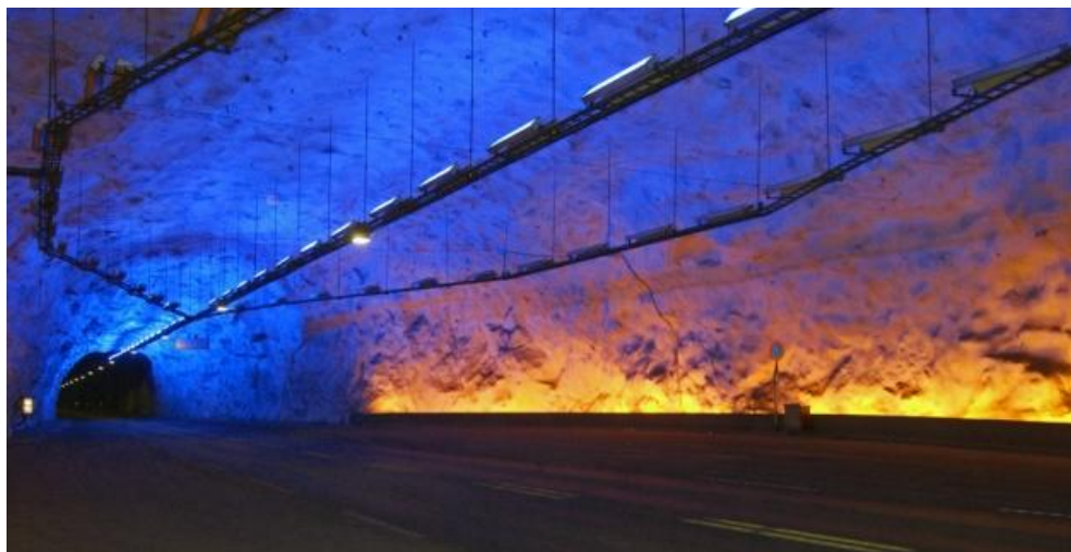
Figure 4.16: Laandertal Tunnel between Bergen and Oslo ( Url - 54 ).
