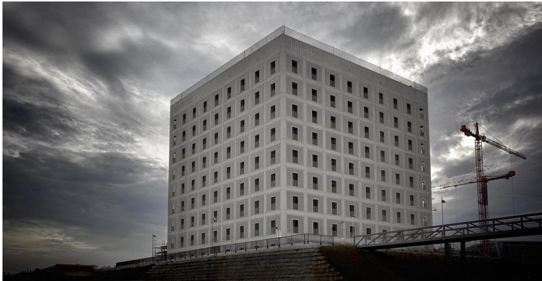
Figure 5.13: Exterior view of Library of Stuttgart (Url - 101).
