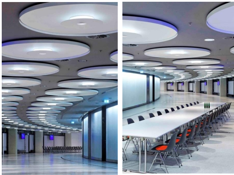
Figure 4.10: Indirect diffuse upward light application of the the business area of Olympic Hall in Munich, by Pfarré Lighting Design (Url - 48).
