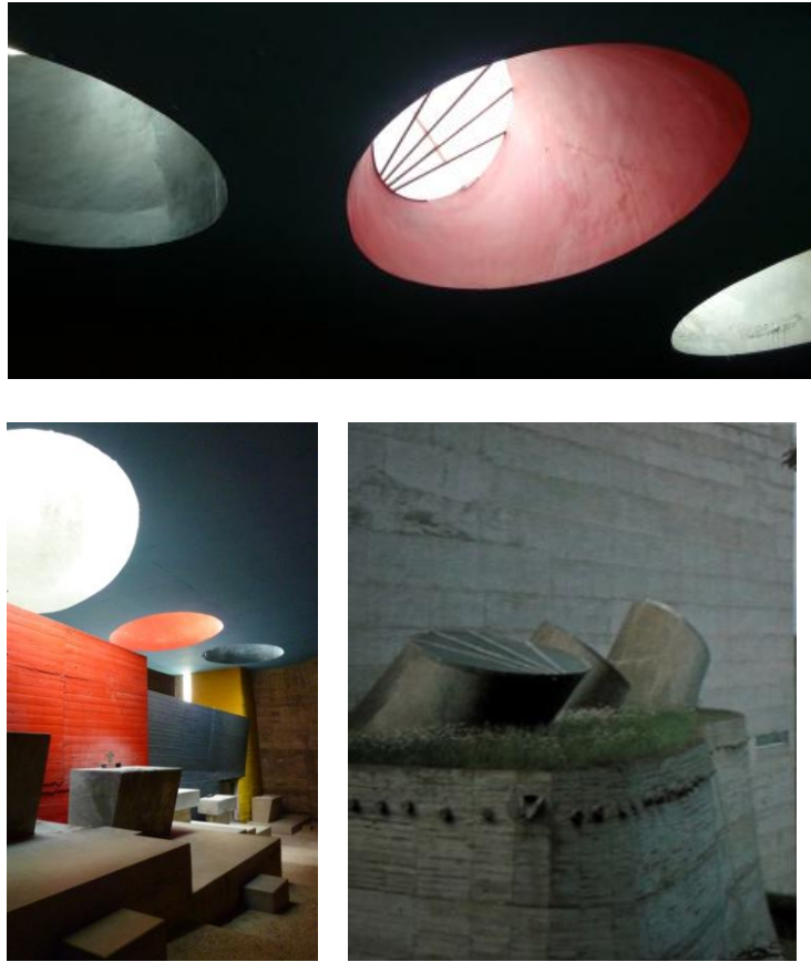
Figure 3.36: Interior and exterior view of rooflights of Corbusier's La Tourette ( M. S. Millet and Barrett, C. , 1996 ).
