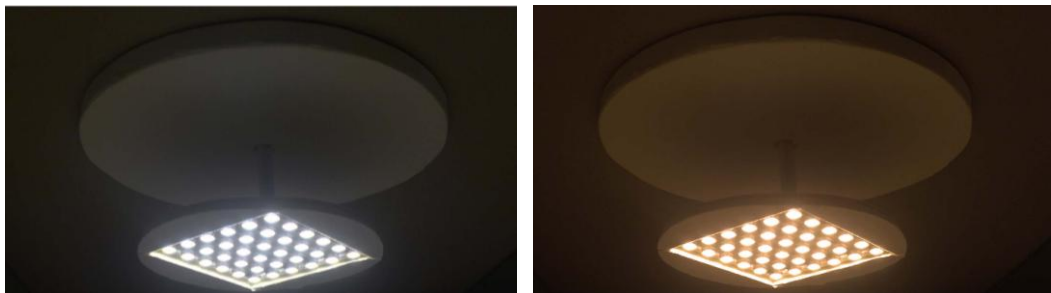
Figure 6.37 : Cold and warm white colour temperature of LED pendant light (Gültekin, 2014)
