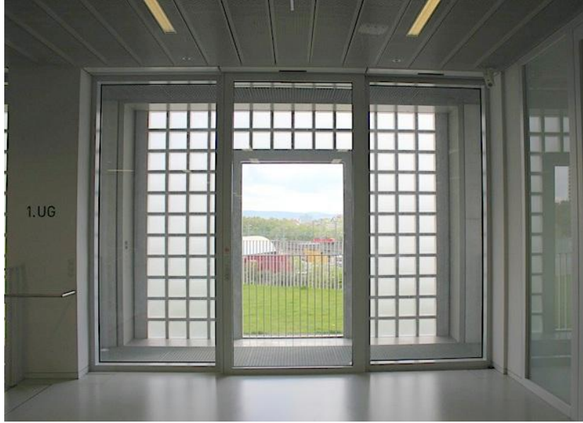
Figure 5.15 : Openings stuffed with glass bricks (Gültekin, 2014).
