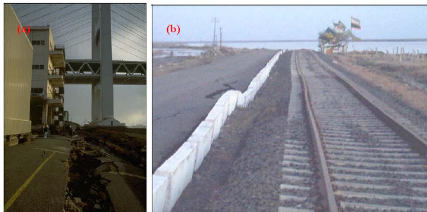
**Figure 4.5 :** Surface observations of lateral spreading at (a) bridge site in 1995 Kobe earthquake (b): Navalakhi port in 2001 Bhuj earthquake, (Bhattacharya,2003)
