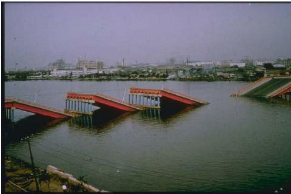
**Figure 4.10:** Failure of Showa Bridge after NISEE, (Hamada, 1992).
