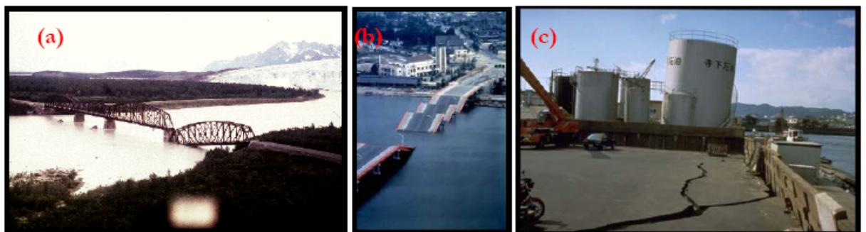
**Figure 4.12:** (a): Piled “Million Dollar” bridge after 1964 Alaska earthquake (USA); (b): Piled “Showa Bridge” after 1964 Niigata earthquake (JAPAN); (c): Piled tanks after 1995 Kobe earthquake (JAPAN), photo courtesy of NISEE.
