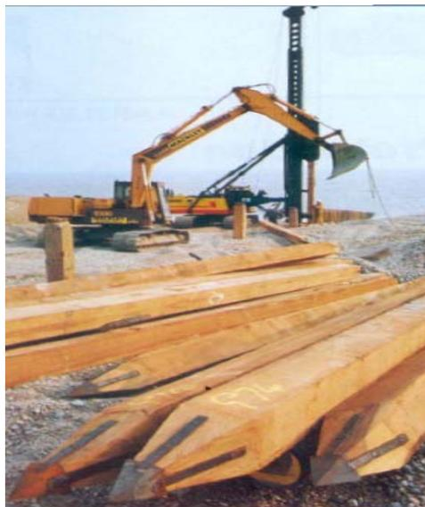
**Figure 2.1:** General view of the timber piles
