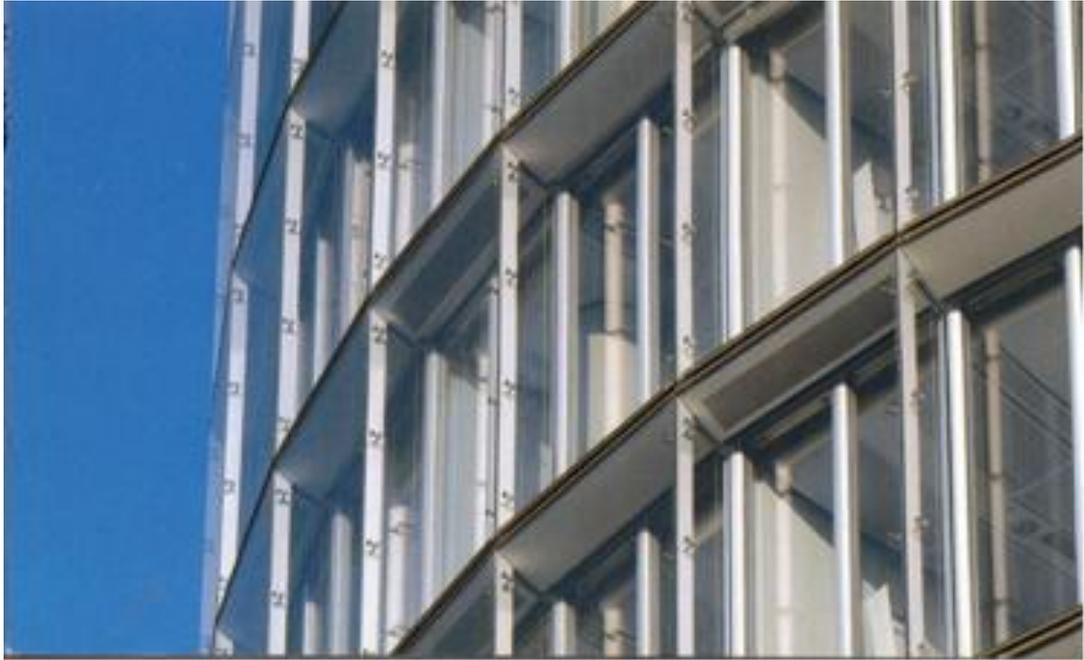
**Figure 3.23 :** Intelligent double layer glass facade, adapted from Höweler (2003).
