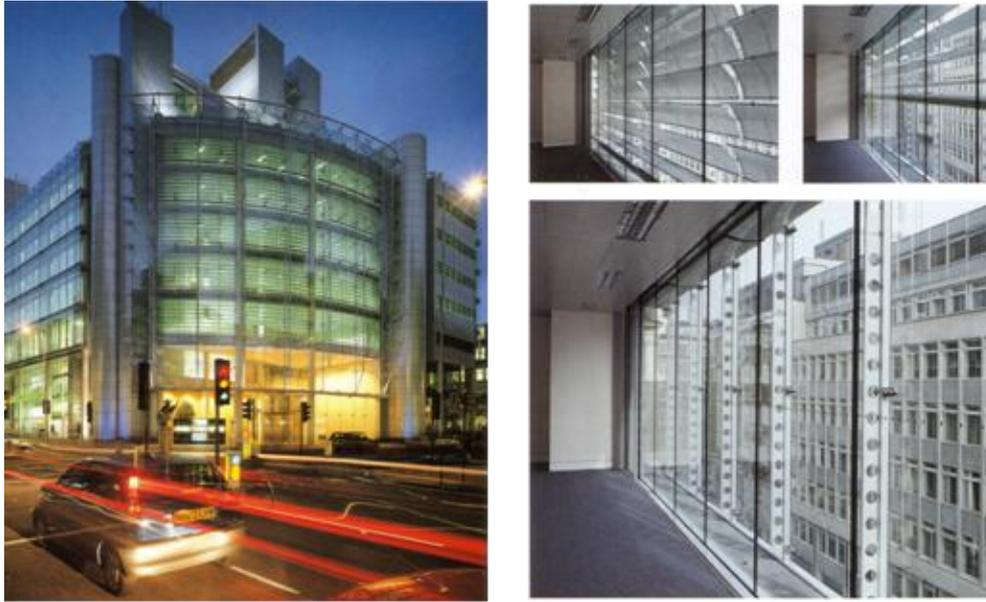
**Figure 4.4 :** The double skin system on the facades of Helicon Building, adapted from Hawkes et al. (2002).
