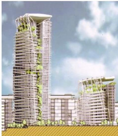
**Figure 3.47 :** The porous cage structure allowing cross ventilation natural daylight, adapted from Höweler (2003).
