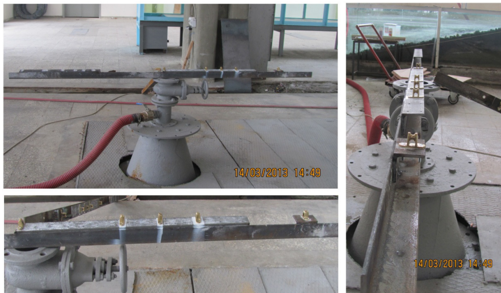
Figure 4.13 : A bottom rail with reels attached prior to installation.
